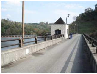
Kyomaru Dam Crest
