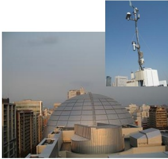
Weather Observation Systems Newly Installed next to the Planetarium of Nagoya City Science Museum
