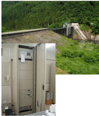
Miyakawa Dam and Telemeter Monitoring System in the Control Office
