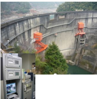
Ayakita Dam and Earthquake Observation System installed in the Office
