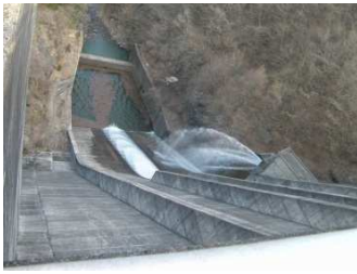
Downstream dam body pictured from dam top(crest of dam)
