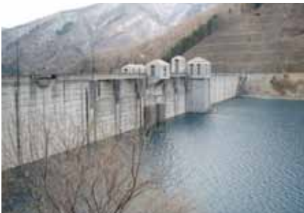
Shimagawa dam at Gunma Pref.
