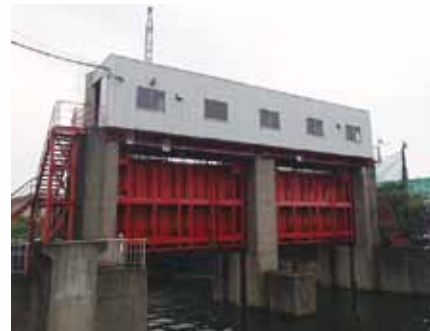
Shirohata Sluice Gate in Chiba Pref.
